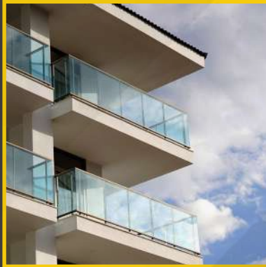
Building Construction Bauindustrie
